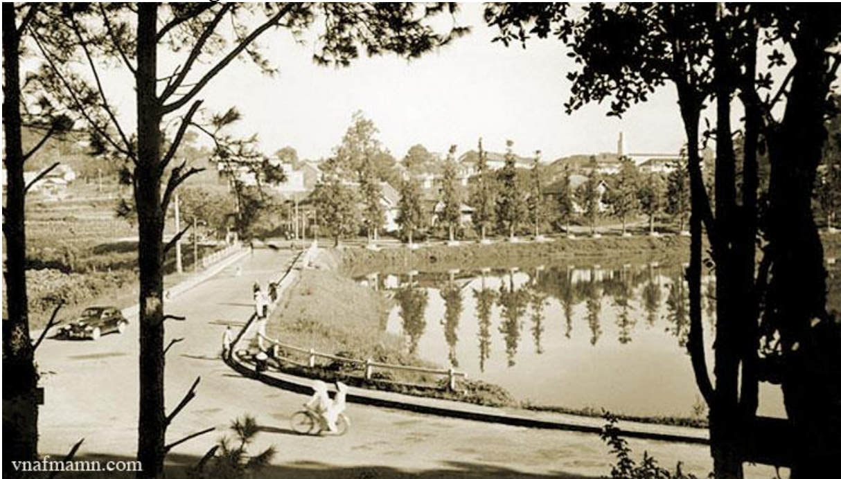
Ong Dao bridge (Dalat, 1957). Same spot but this photo is a different shot from the previous one.
